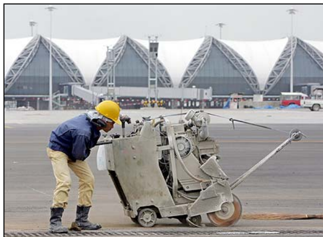
Balanced pavement saw
