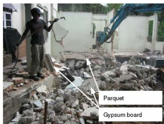
Illustration 15: Crushing the structure, foreign material in the debris
